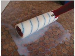
11. After the grout has fully cured, finish the installation of the Jelinek Cork Mosaic by evenly and thoroughly applying two additional coats of water-based polyurethane in the same manner as in step 7. It is extremely important that the grout is dry and also that the entire area has been covered with the polyurethane to ensure a complete seal. Failure to do so will result in discolouration of the grout.
