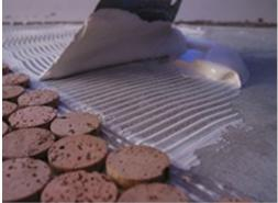
**Note:** Tiles can also be adhered using a water based Acrylic Mastic as this image represents.
